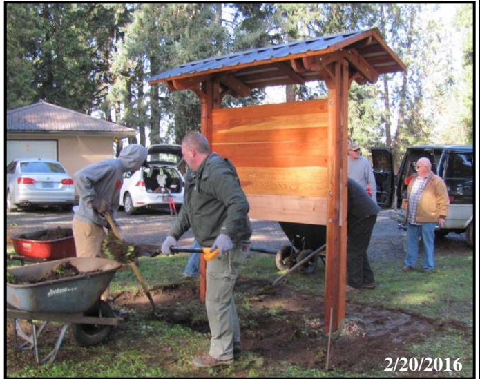
INSTALLING THE KIOSK IN MEMORIAL SQUARE
